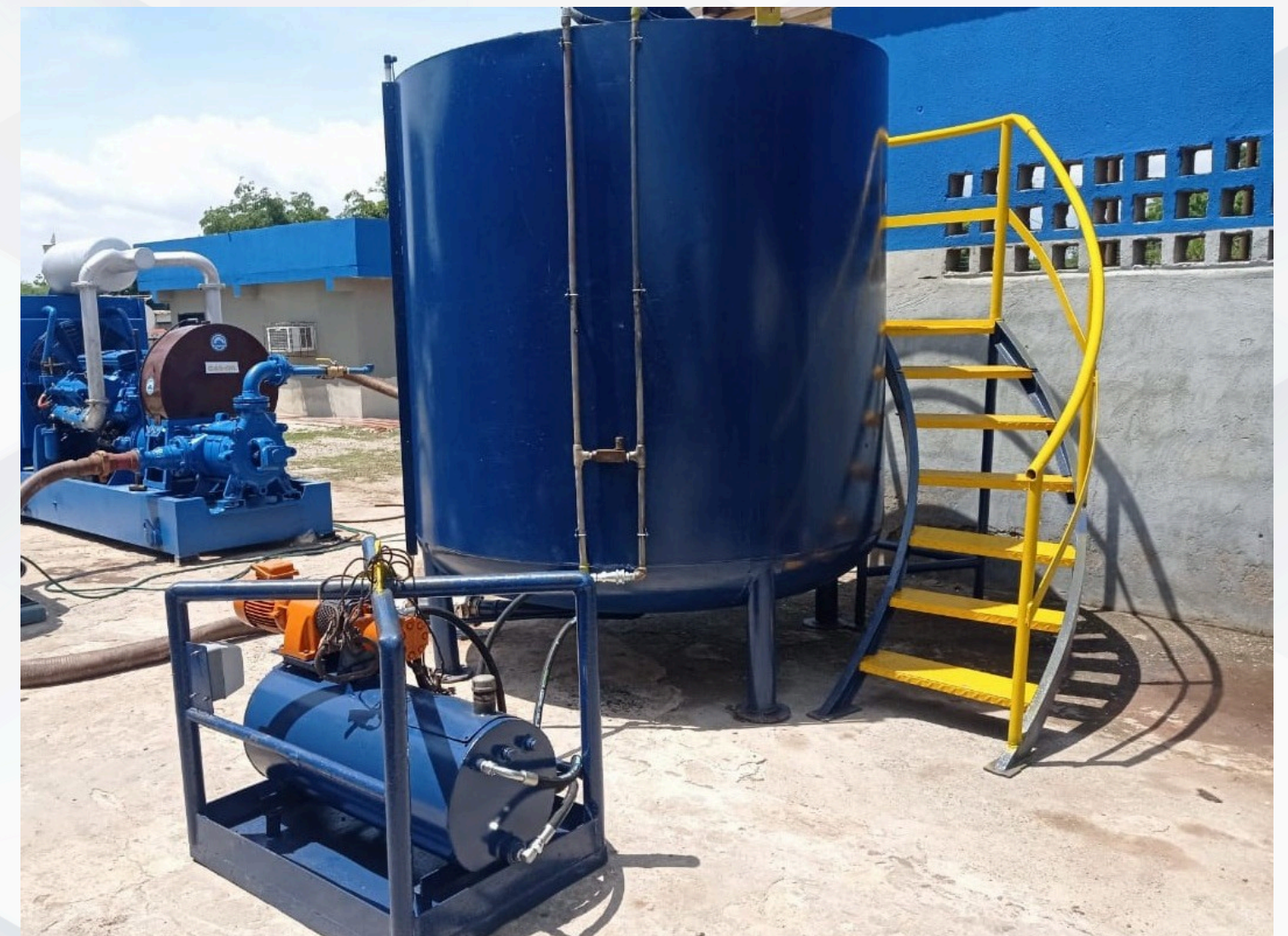
Assembly on site: tank, agitator and pumping unit.
